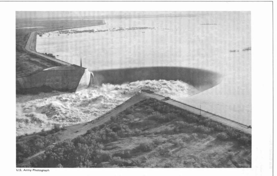
Figure 24--Aerial View of the Spillway of the Marte Gomez Reservoir on the Rio San Juan Discharging About 150,000 cfs
