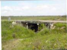
18. Upstream side of bridge on CR 67 over North Hapt Creek.
