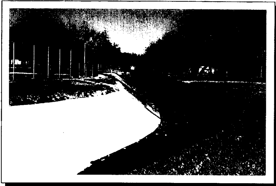
Figure III-11a - Typical Concrete Section in Lower PEC-4 Channel
