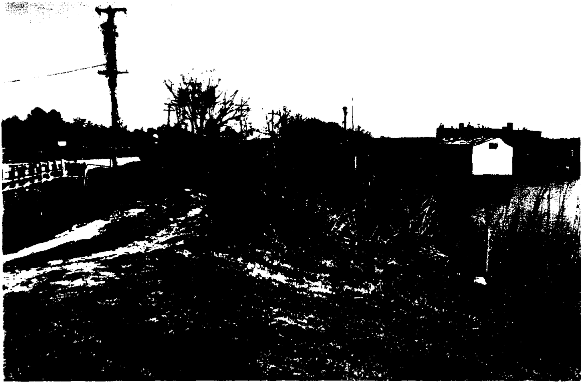
PHOTO III.3 Existing Levee Near Coopers Pump Station
