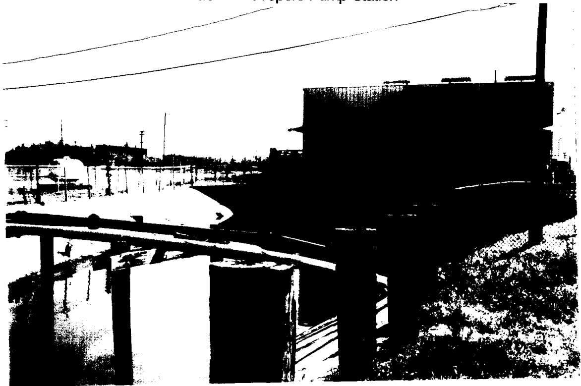
PHOTO III.6 Coopers Pump Station
