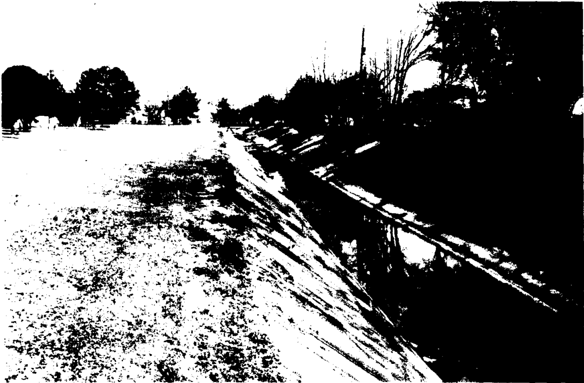
PHOTO III.13 View of Concrete Lined Channel D/S of 37th St.
