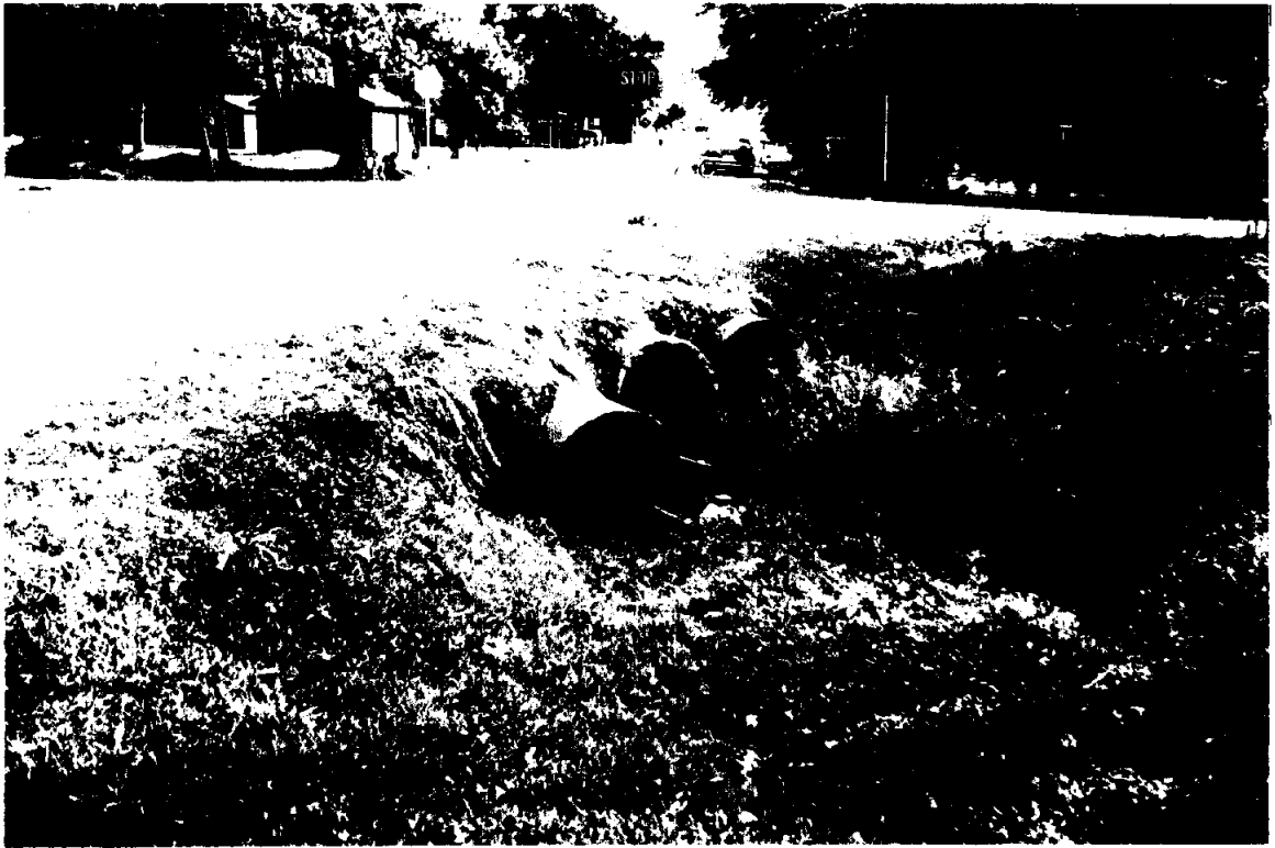
PHOTO III.9 View of Tanglewood Culverts
