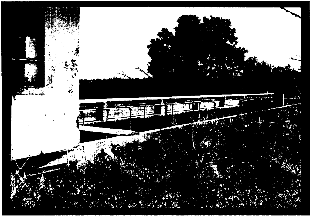
Old Cisco Activated Sludge Plant
