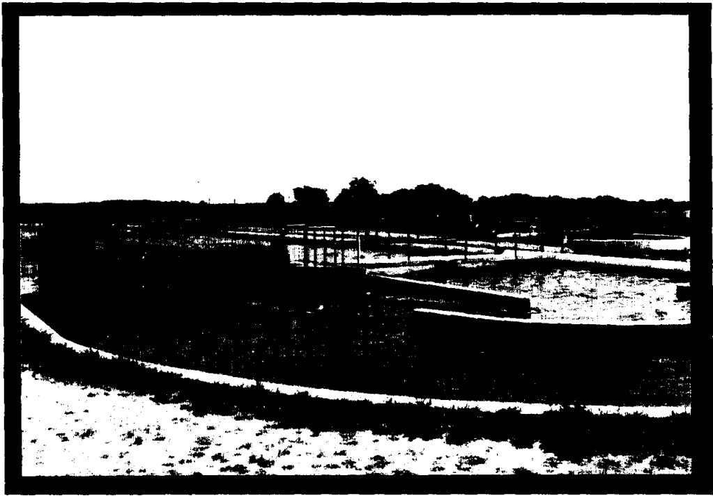
Eastland Oxidation Ditch Plant
