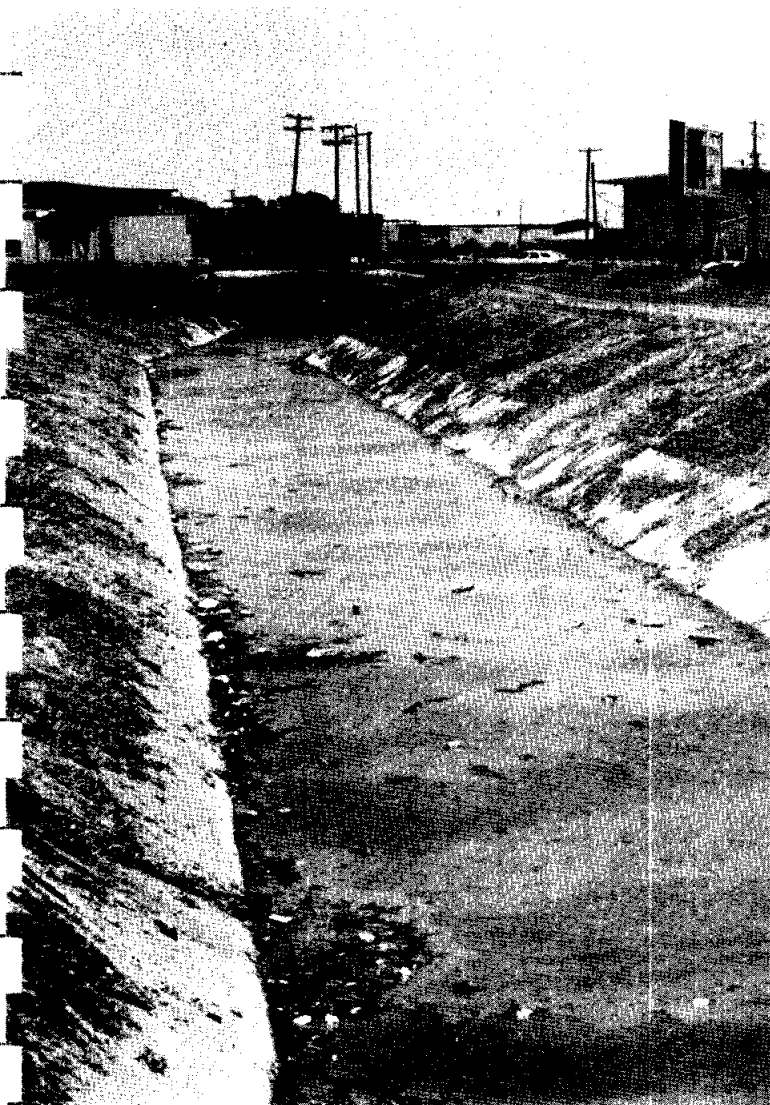
NORTH MAIN DRAIN North Main Drain After Cleanout, Summer 1986
