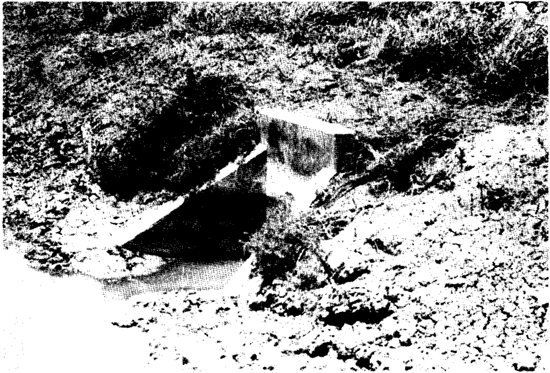
AIRPORT DRAINAGE Airport Drainage Outlet Headwall Note Sediment Line on Headwall After Recent Ditch Cleanout
