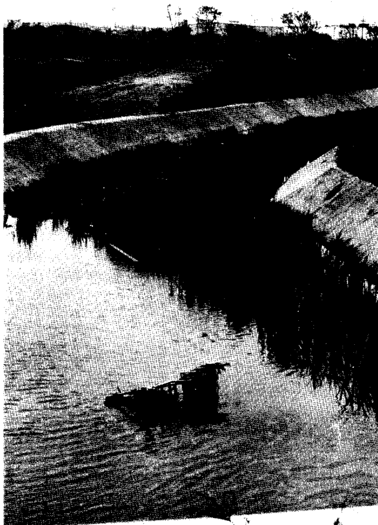
NORTH MAIN DRAIN North Main Drain a Few Months After Cleaning, Fall 1986
