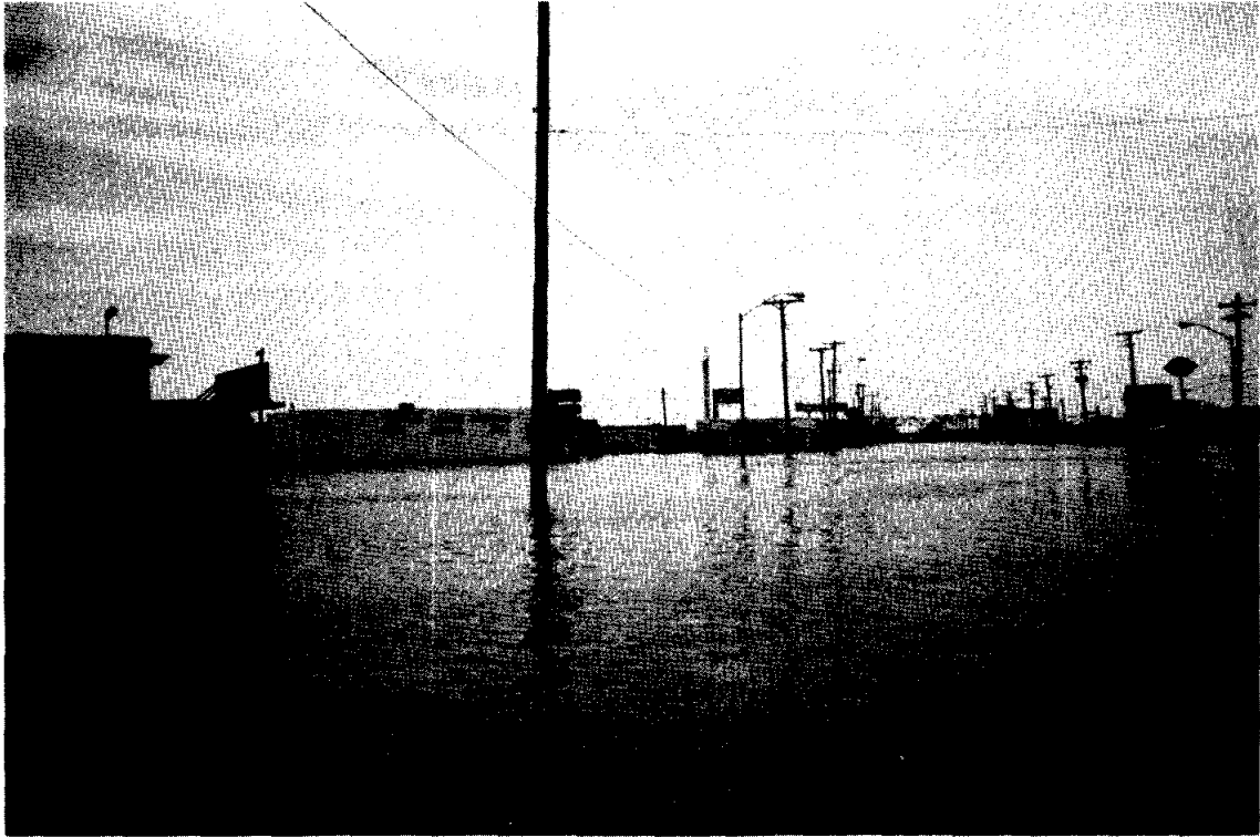
RESACA DE LA GUERRA Flood Conditions on Boca Chica Boulevard, September 1984 Flooding From Main North Drain and Resaca de la Guerra Looking West From Four Corners Area
