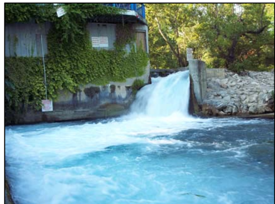
Figure 17. Typical Spring Lake Spillway Discharge
