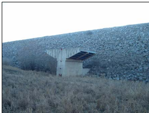
Figure 5. NRCS No. 5 Primary Outlet (typical of all five NRCS reservoirs)
