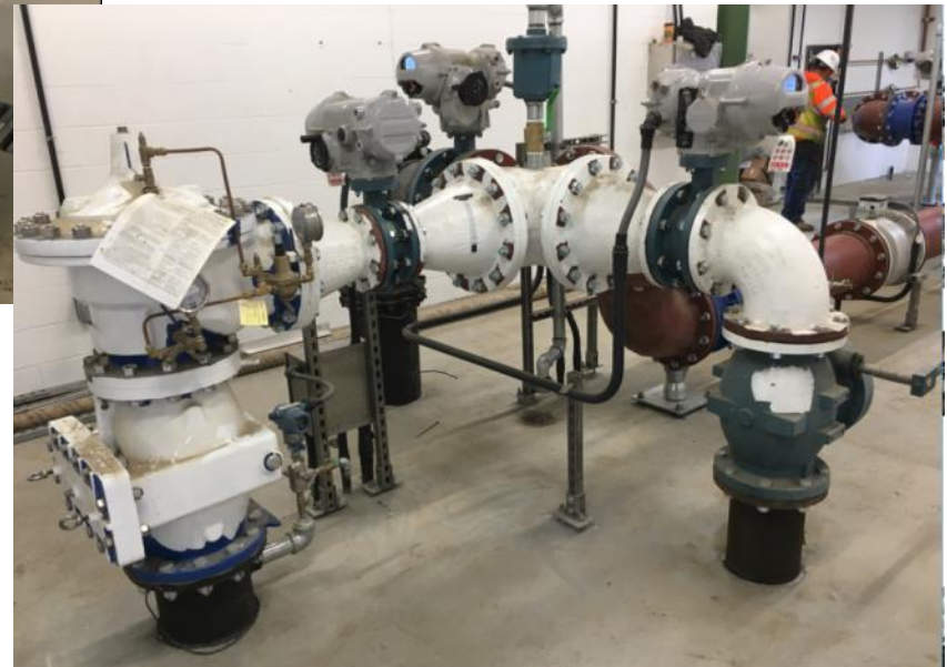
View at Strainer/PRV End of Wellhead Piping
