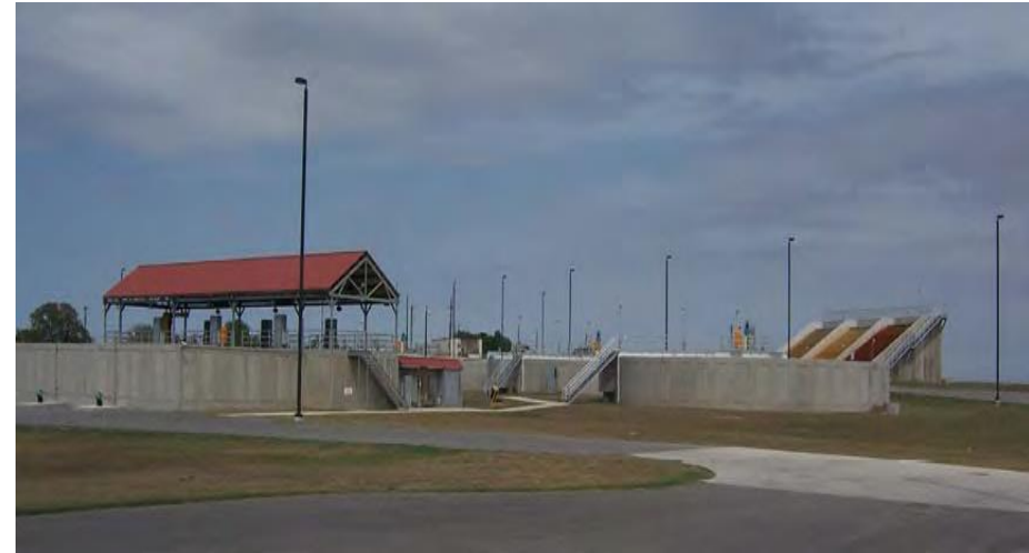
SAWS Twin Oaks Water Treatment Plant at the ASR Wellfield, 2006
