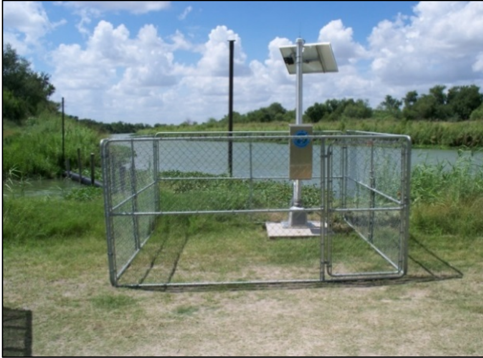
Figure 5. CAMS 789, Rio Grande at the Harlingen Irrigation District (ID) Diversion. View downstream with the irrigation diversion to the left and the Rio Grande flowing from right to left. Photo by TCEQ.
