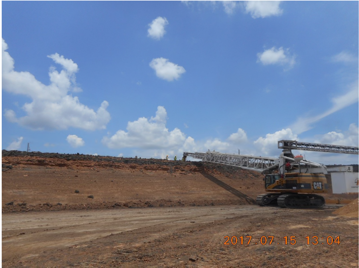
Figure 4-7. Placement of Chimney Drain Cap
