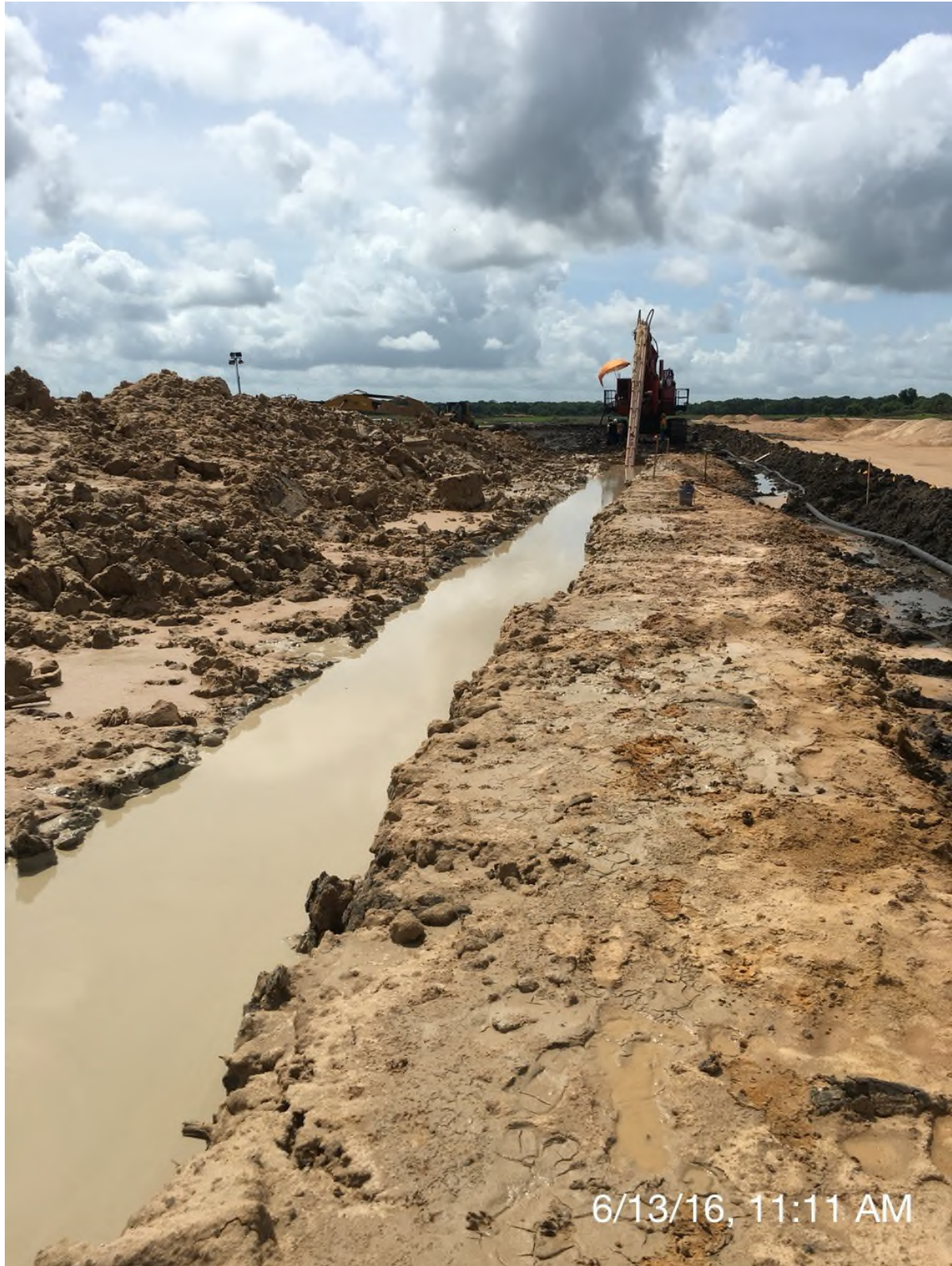
Figure 3-20. Soil-Bentonite Cut-off Wall Installation
