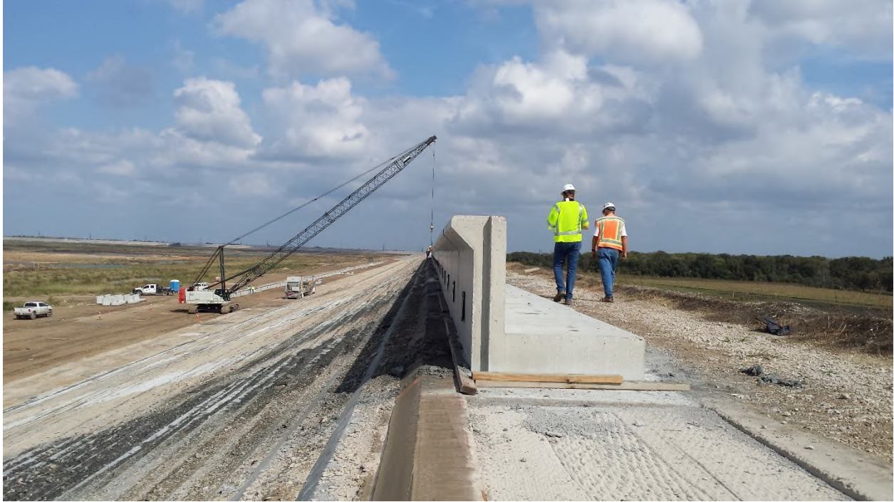
Figure 4-17. Wave Wall Panels Placed on the Embankment Crest
