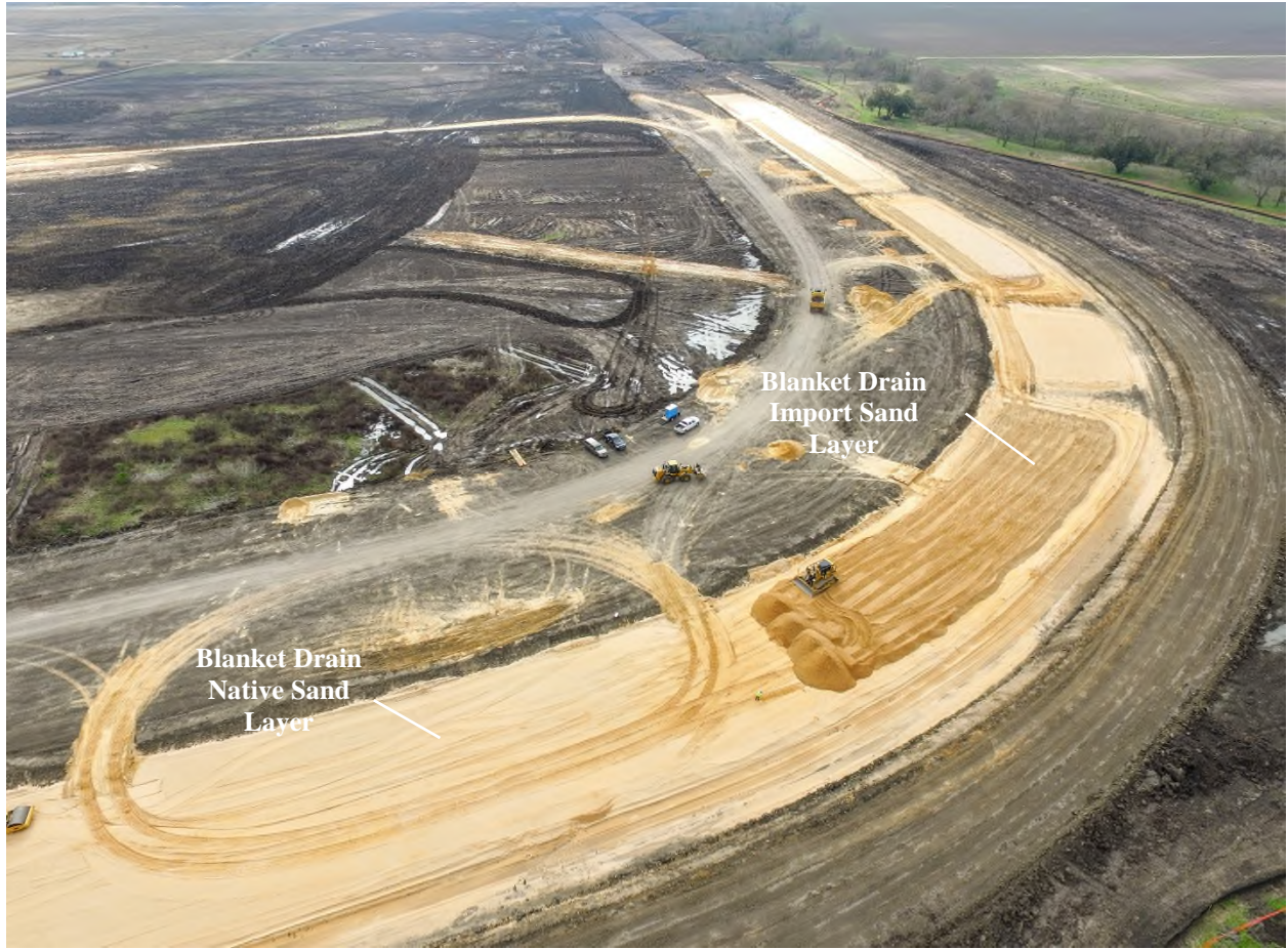
Figure 3-15. Blanket Drain Installation, Northwest Corner of Embankment, Looking South
