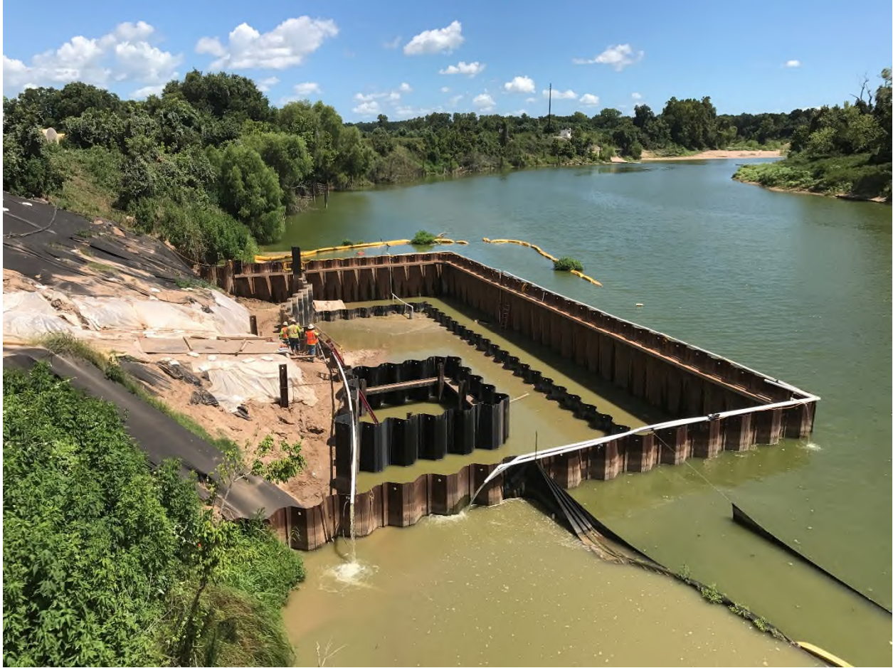
Figure 4-24. Permanent Sheetpile Installation Inside the Cofferdam on the River
