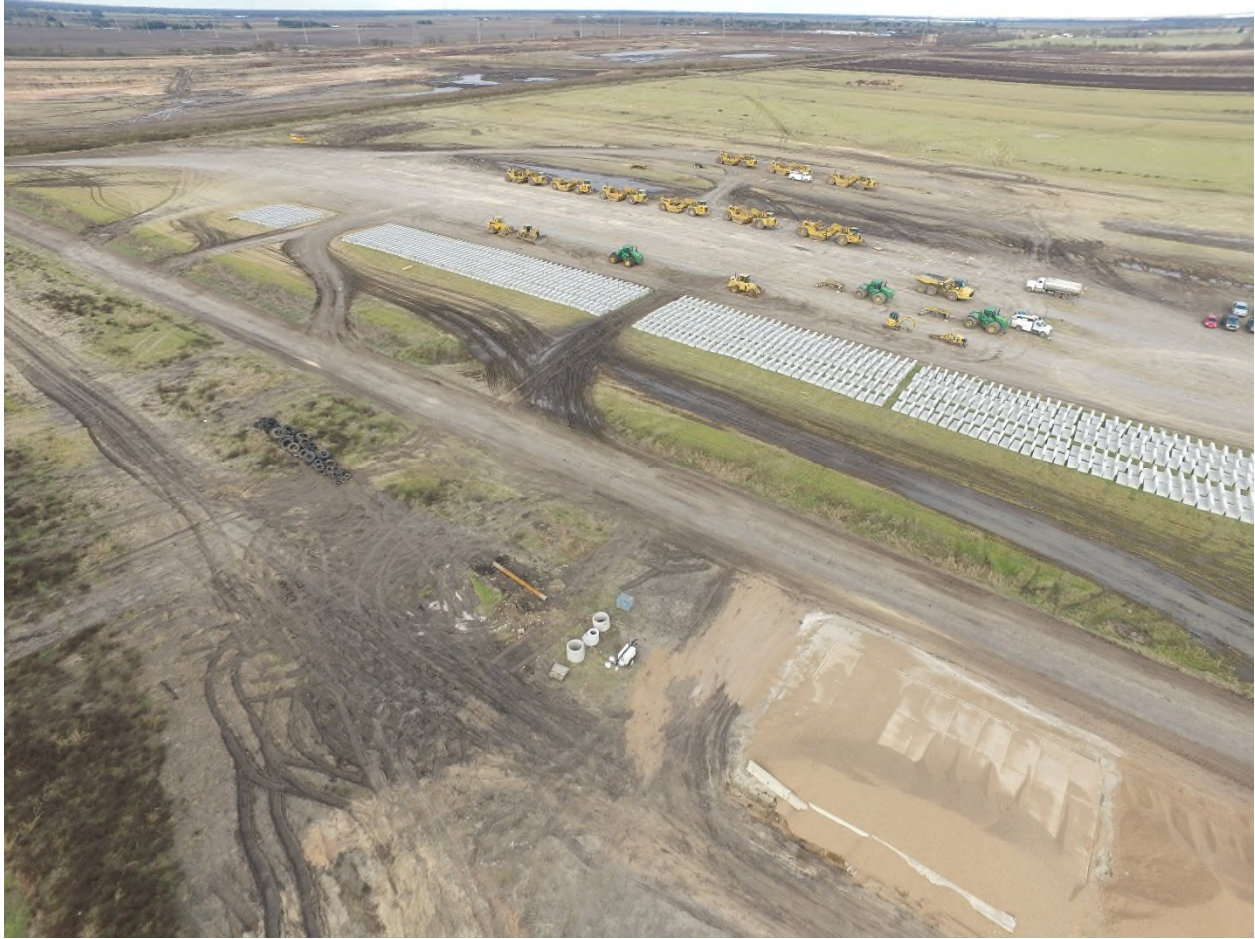
Figure 4-11. Wave Wall Panels Stored On-site on OCR Interior
