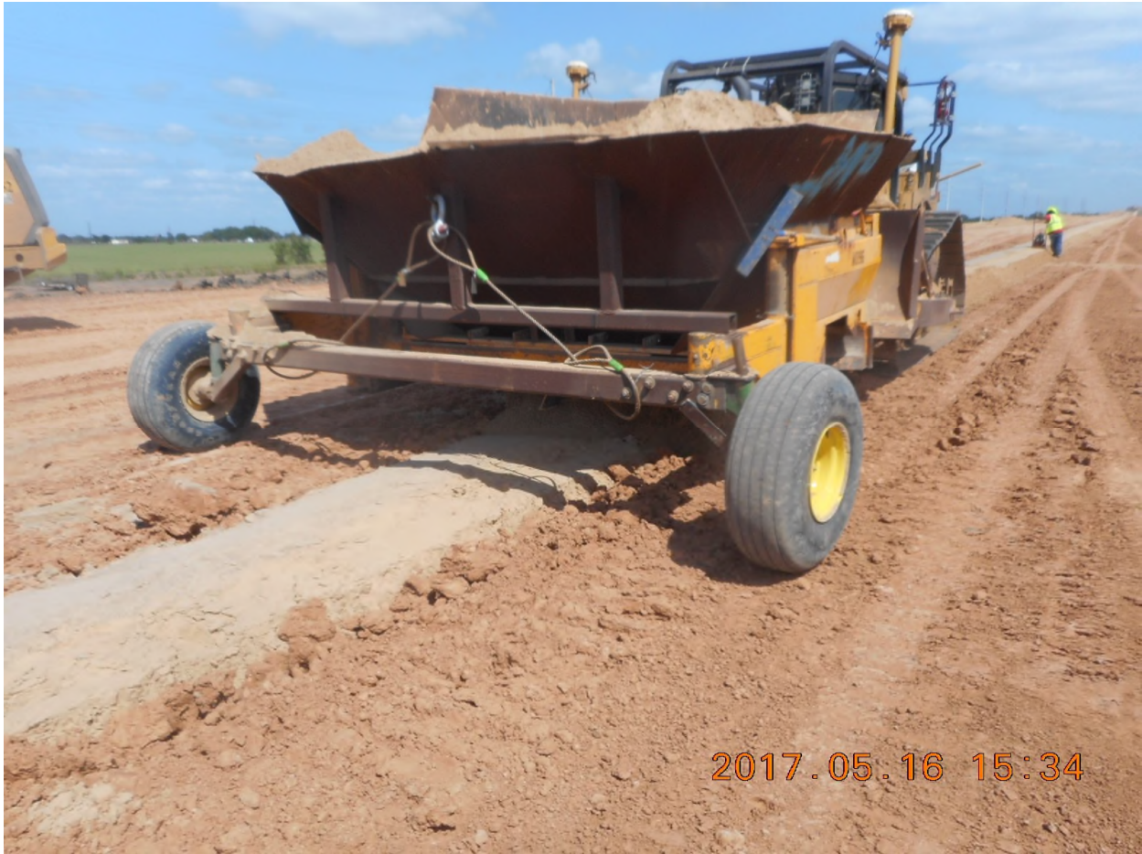
Figure 4-5. Flotation Tires Added to Rock Spreader Box
