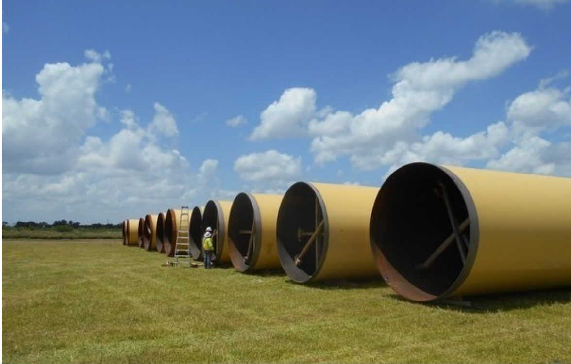
Figure 3-10. OCR Inlet/Outlet Pipe Sections Awaiting Installation
