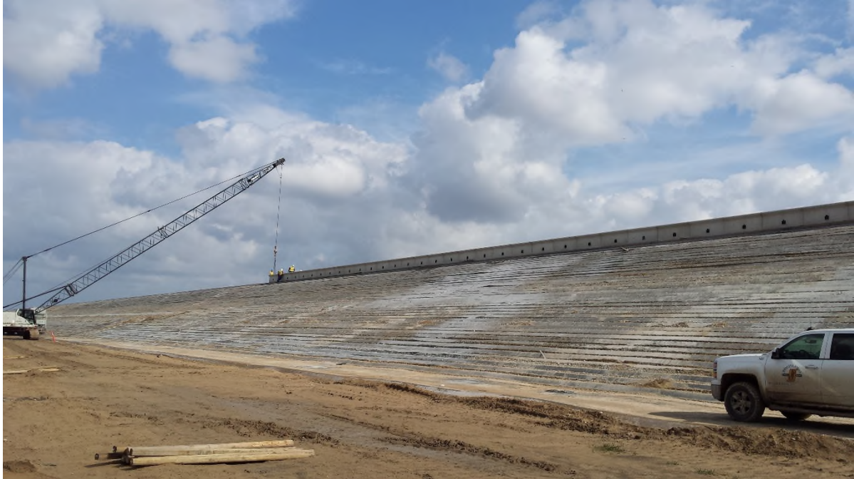
Figure 4-12. Crane Lifts Wave Wall Panels to Embankment Crest
