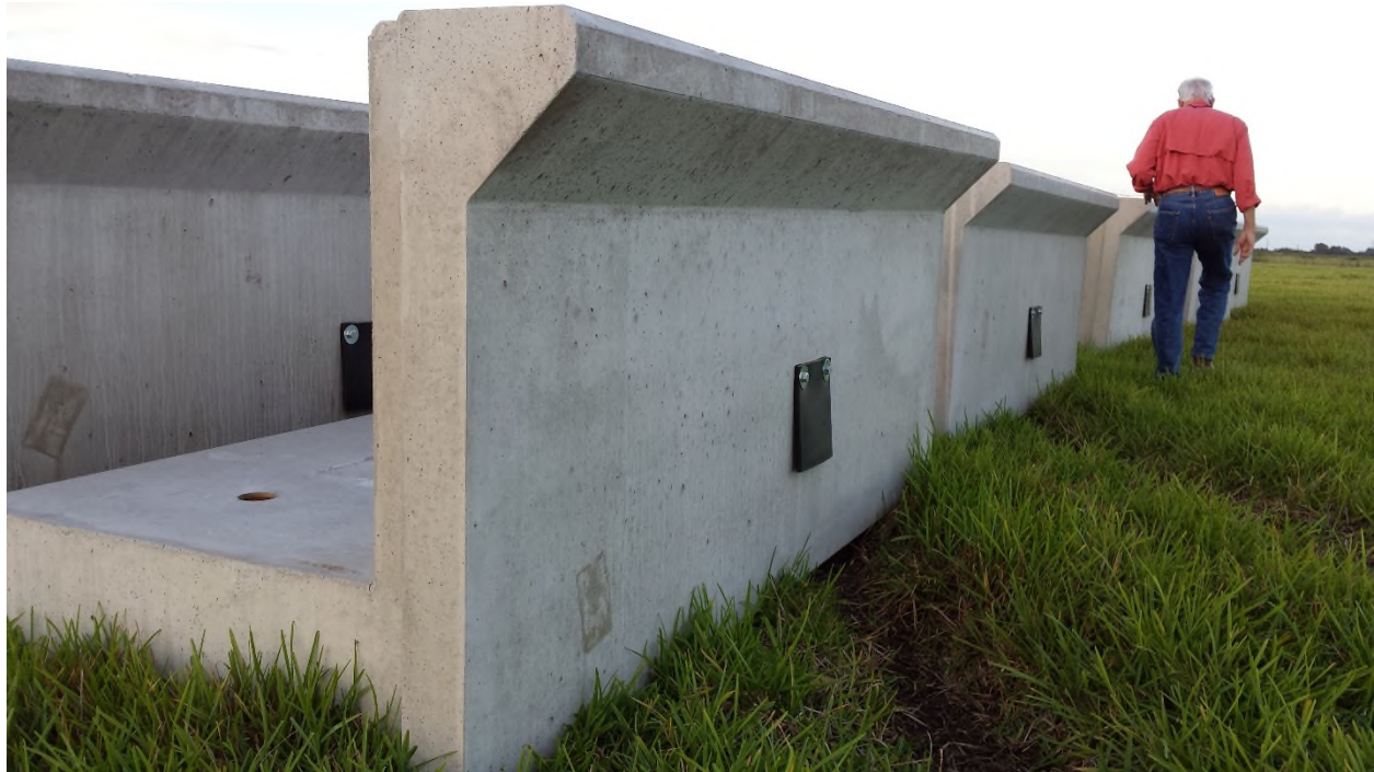
Figure 4-8. Wave Wall Segments Stored and Awaiting Placement
