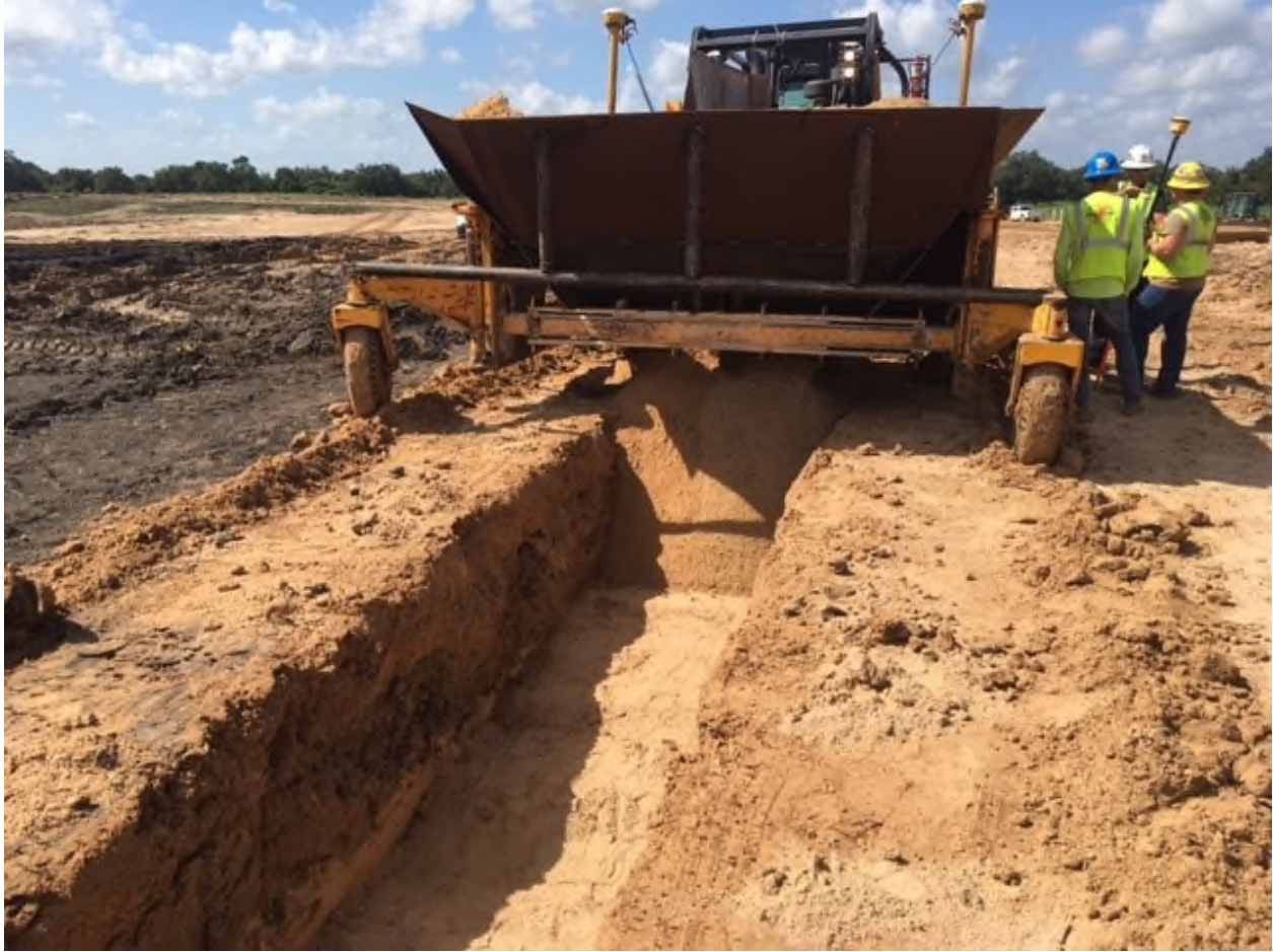
Figure 4-4. GPS Equipped D6 Dozer and Modified Rock Spreader
