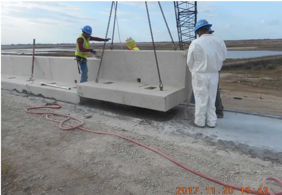
Figure 4-12. Crane Lifts Wave Wall Panels to Embankment Crest
