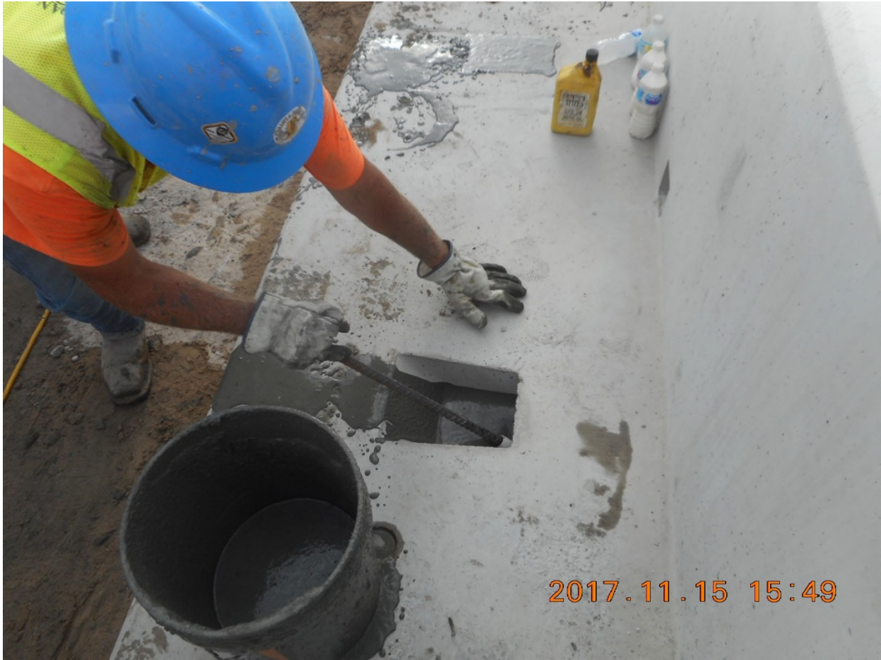
Figure 4-15. Steel Anchors are Placed in Each Drilled Hole
