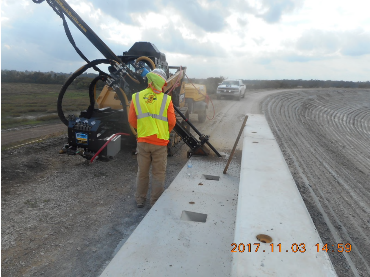
Figure 4-14. Holes are Drilled into the Soil Cement Steps
