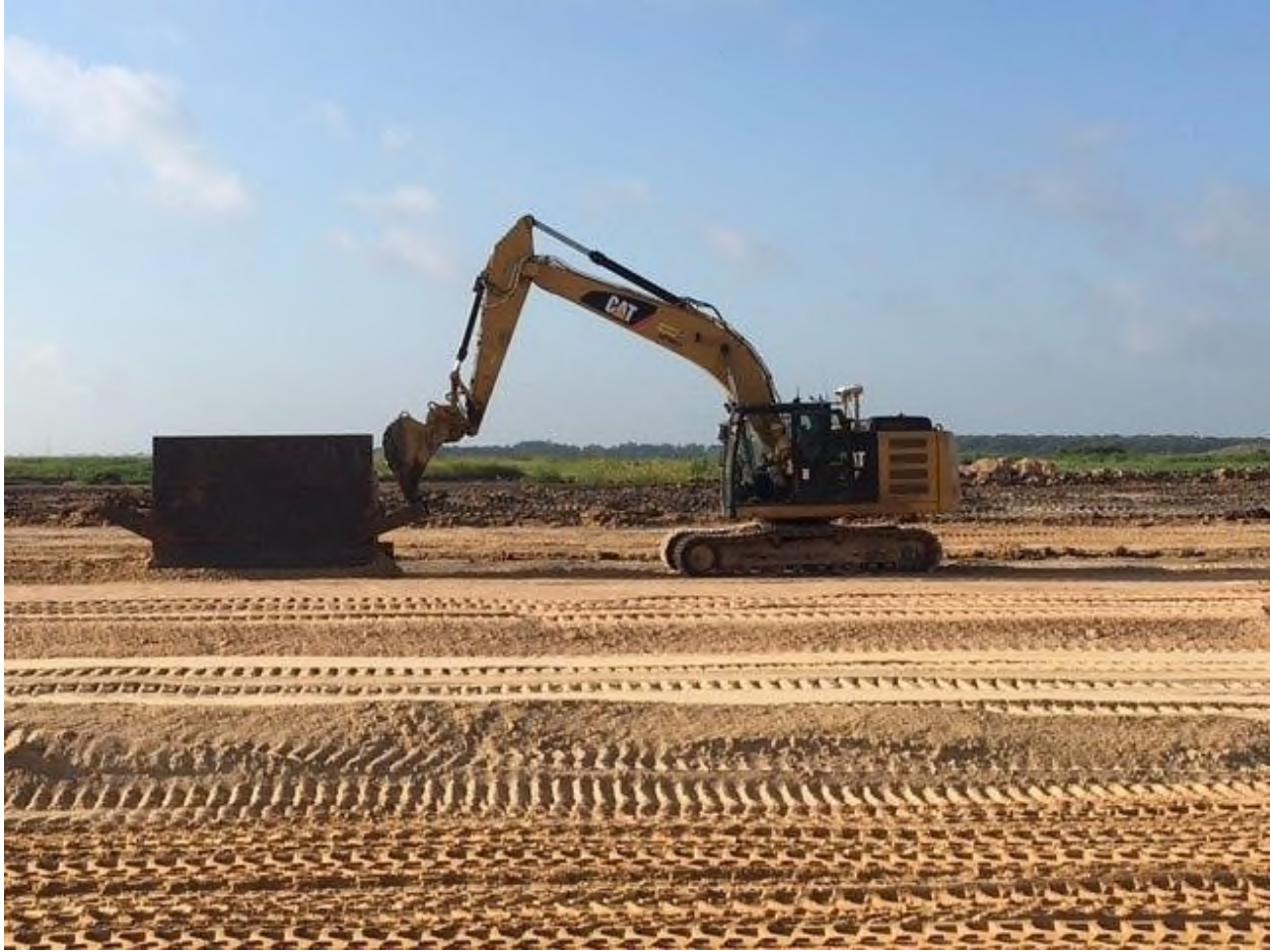
Figure 4-3. Divider Box Pulled along Trench by Excavator
