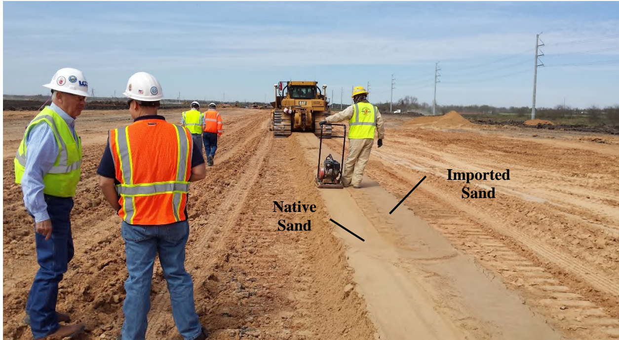
Figure 4-6. Chimney Drain Sands Placement
