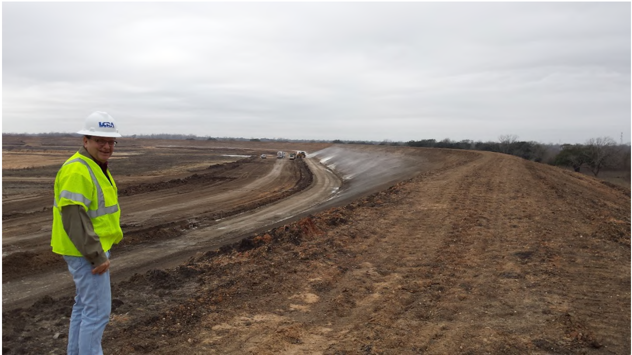
Figure 3-14. Top of Northwest Embankment Corner, Looking South
