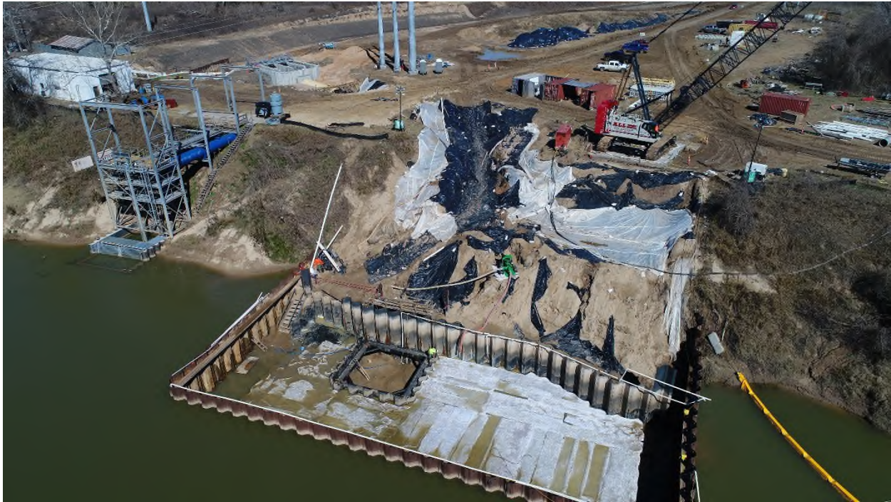
Figure 4-21. Aerial View of River Return Structure Construction at River
