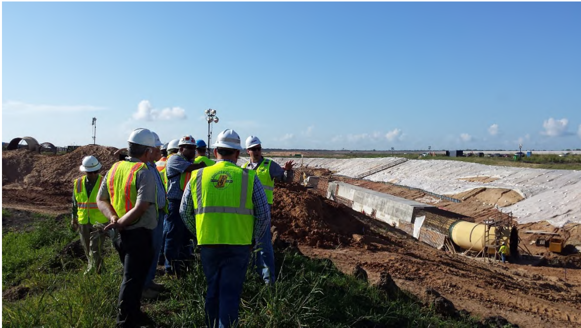
Figure 3-9. OCR Inlet/Outlet Construction
