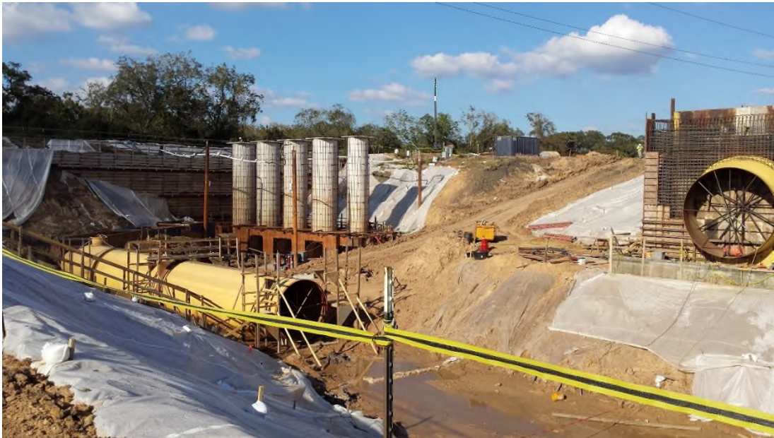
Figure 3-8. Relift Pump Station Construction
