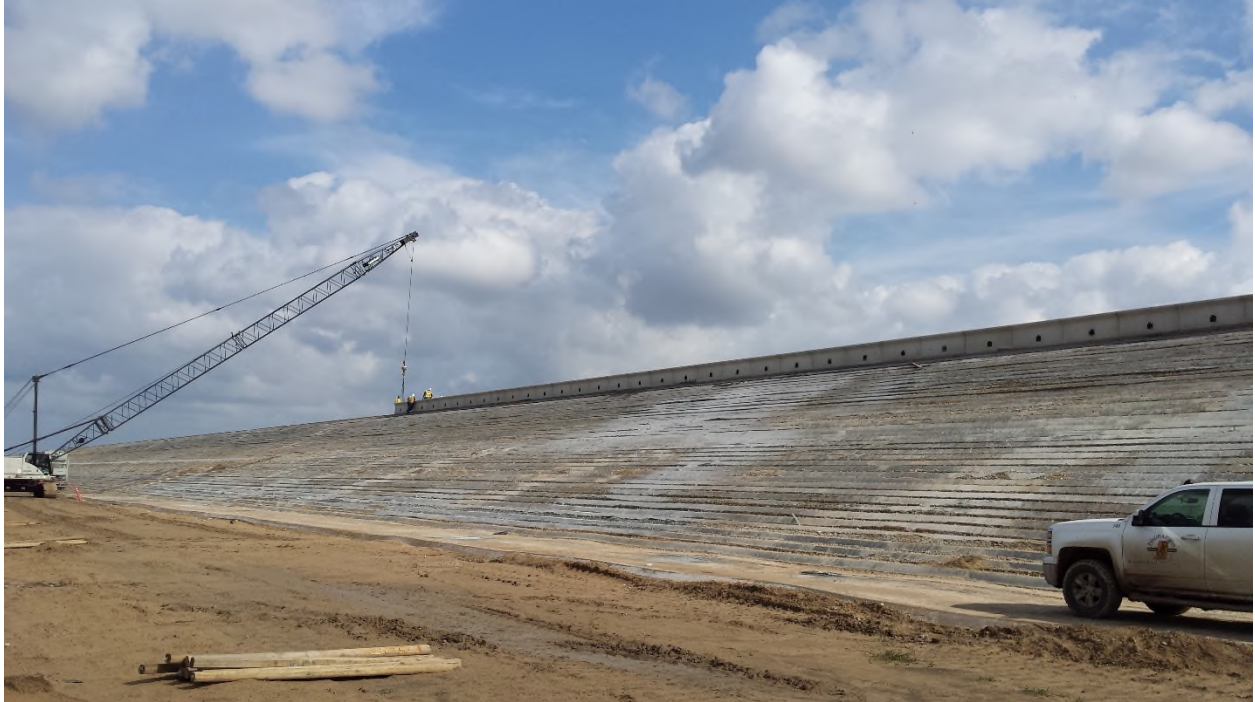
Figure 3-18. Soil Cement Steps and Wave Wall Placement on Embankment Top
