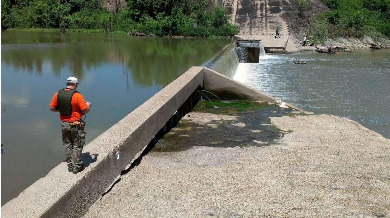
Figure 3-24. Lane City Dam, Right (West) River Bank Looking East
