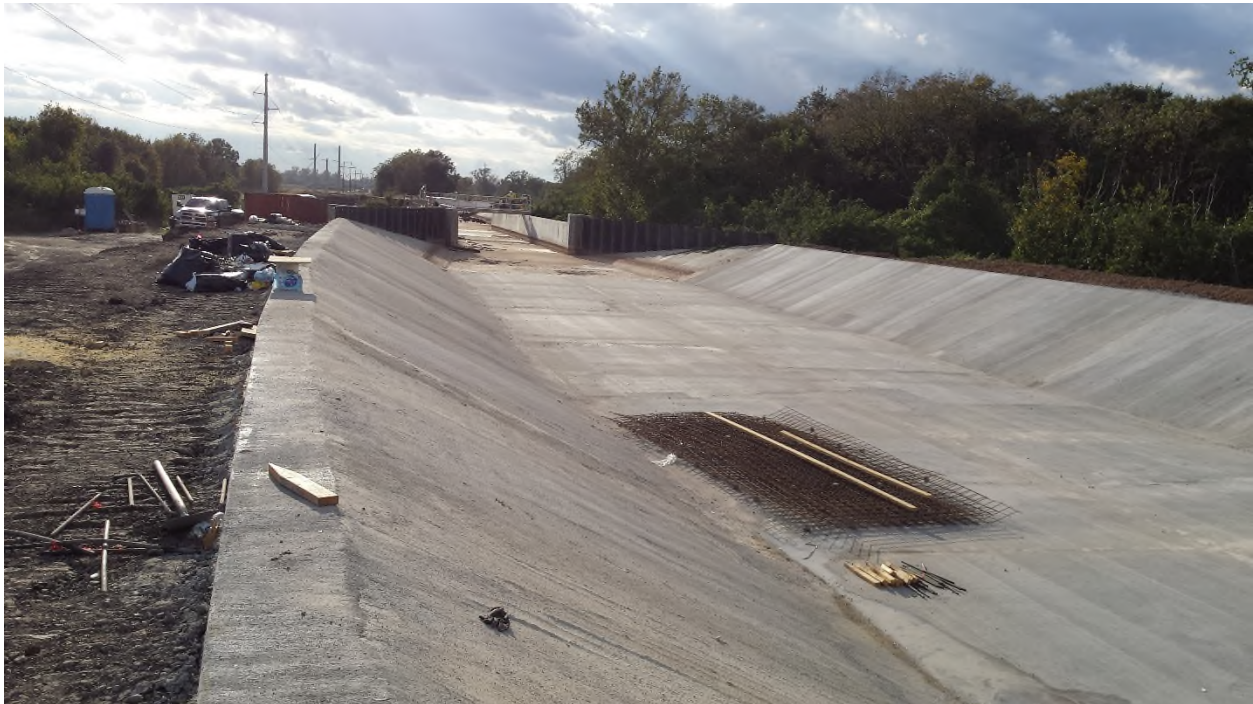
Figure 3-5. Canal Lining Near Flume Over Jarvis Creek
