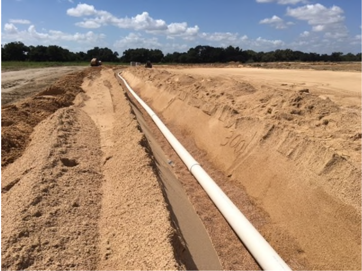
Figure 3-17. Toe Drain Installation
