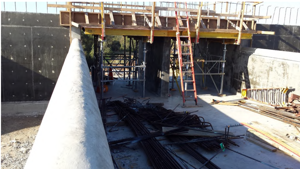
Figure 3-22. Spillway Crest Construction Looking West from Inside Reservoir
