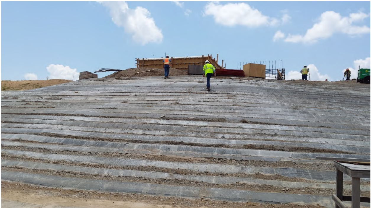
Figure 3-19. Soil Cement Steps During Spillway Construction
