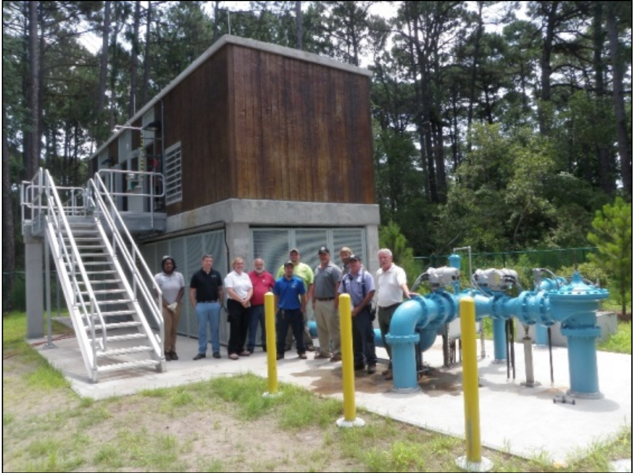
Figure 4-12 ASR Well on Platform at Hilton Head Island, South Carolina
