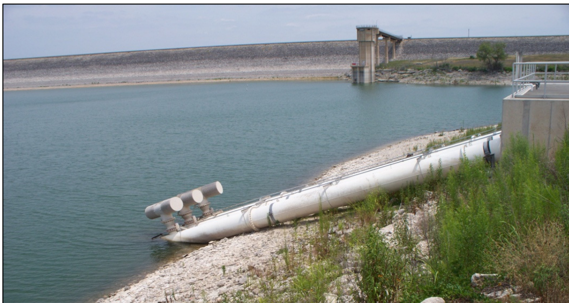
Figure 7-2: Photograph of Inclined Can Intake Structure
