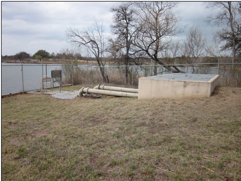
Figure 7-3: Photograph of Wet Well Intake Structure
