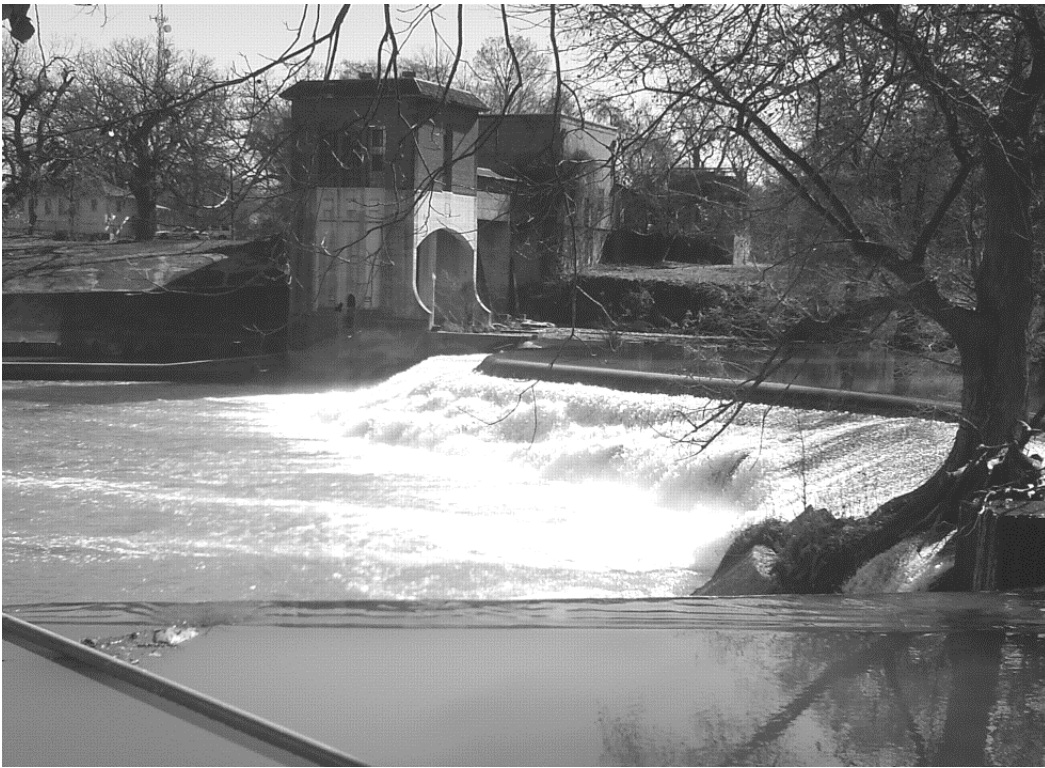
Figure 22. Hydroelectric dam on the Guadalupe River at Seguin in zone 9.
