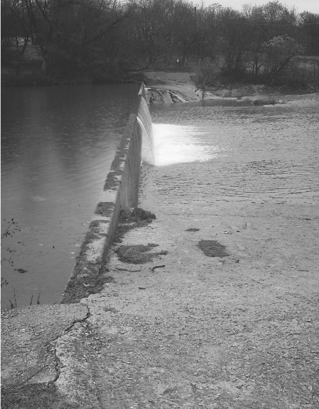
Figure 8. Low-head dam near Center Point.
