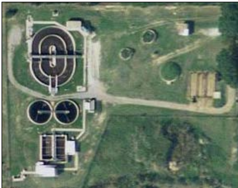
Figure 1.8 Aerial View of the Van Alstyne WWTP
