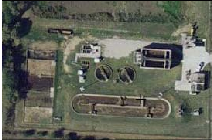
Figure 1.1 Aerial View of Celina WWTP
