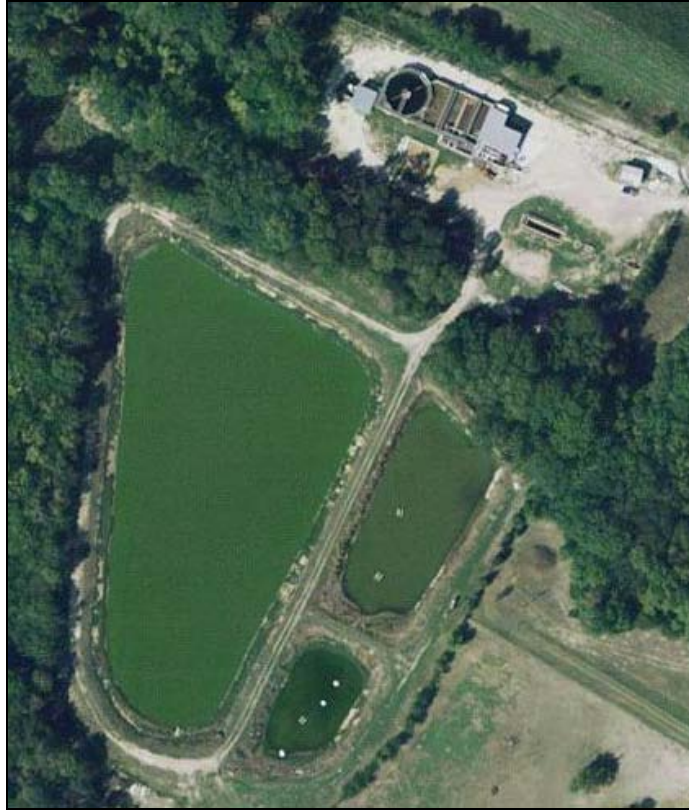
Figure 1.16 Aerial View of the Anna WWTP
