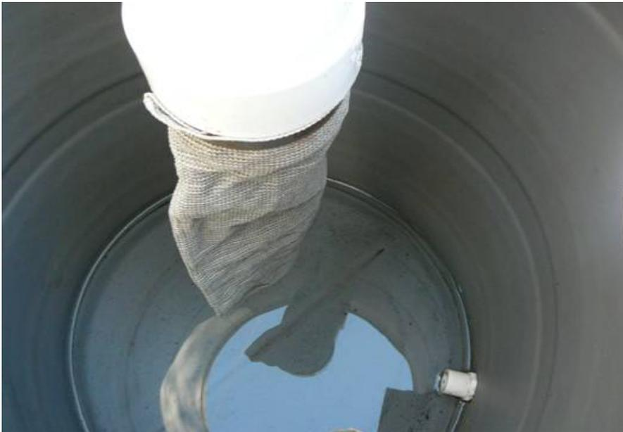
Sock filter to remove coarse debris.
