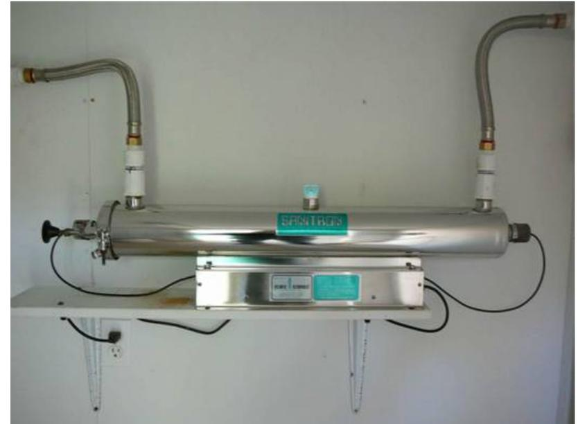
Ultraviolet filters for potable water system.
