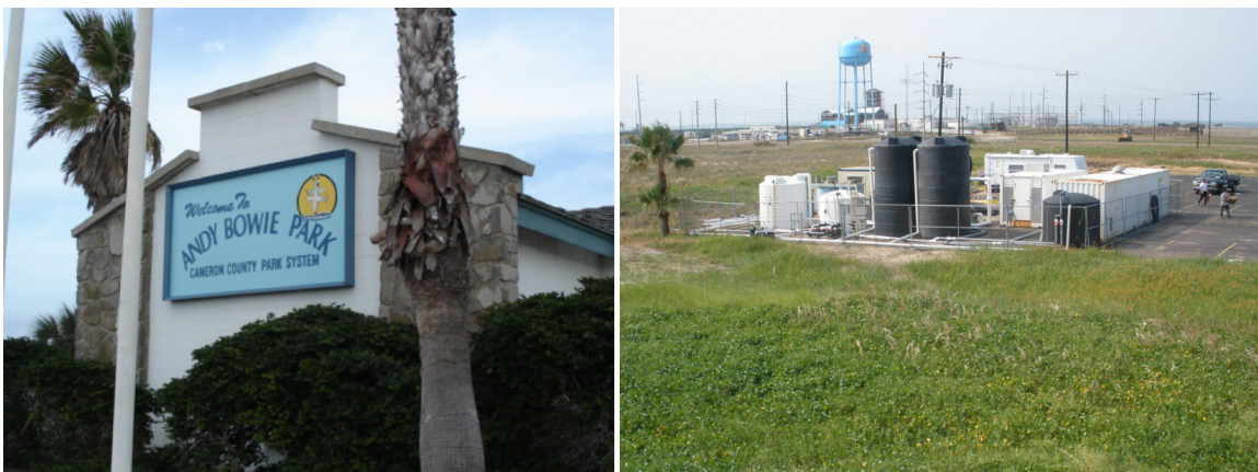
Figure II-4: Andy Bowie County Park entrance (left) and pilot site (right).
