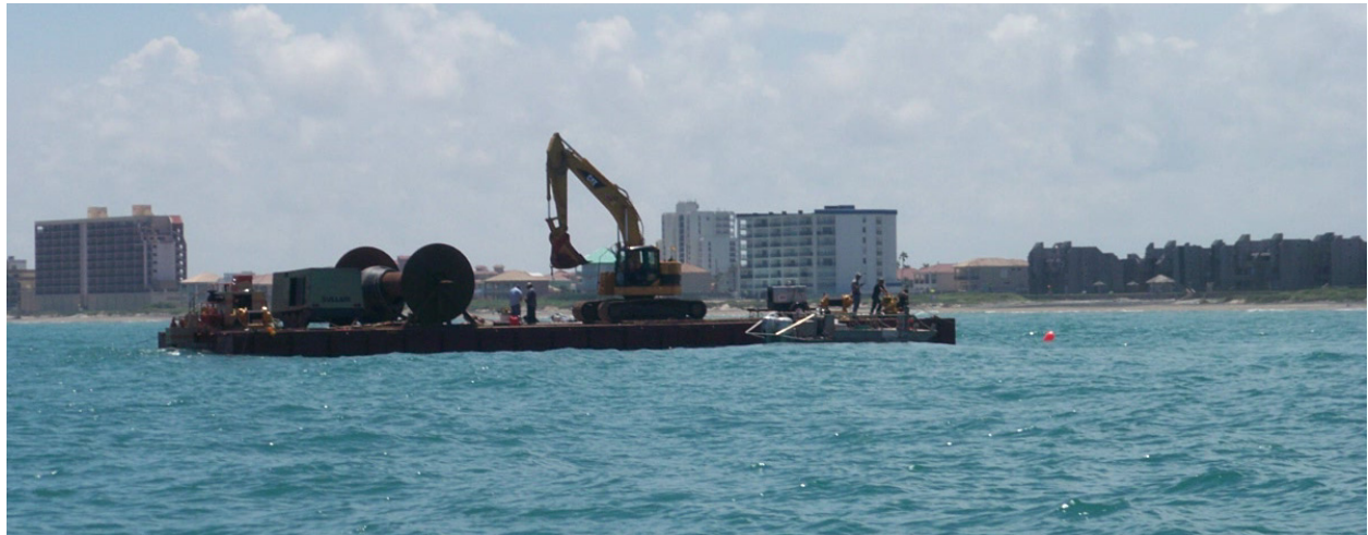
Figure II-5: Janco Directional Drilling installing intake.
