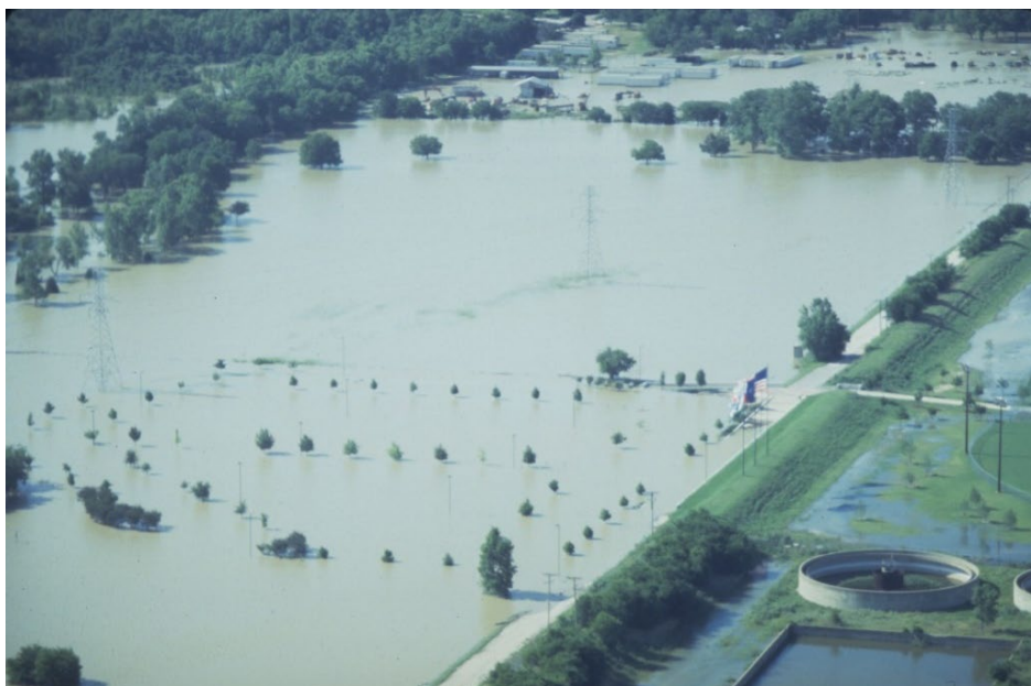
Figure 1.22: Flooding, Trinity River Levees
