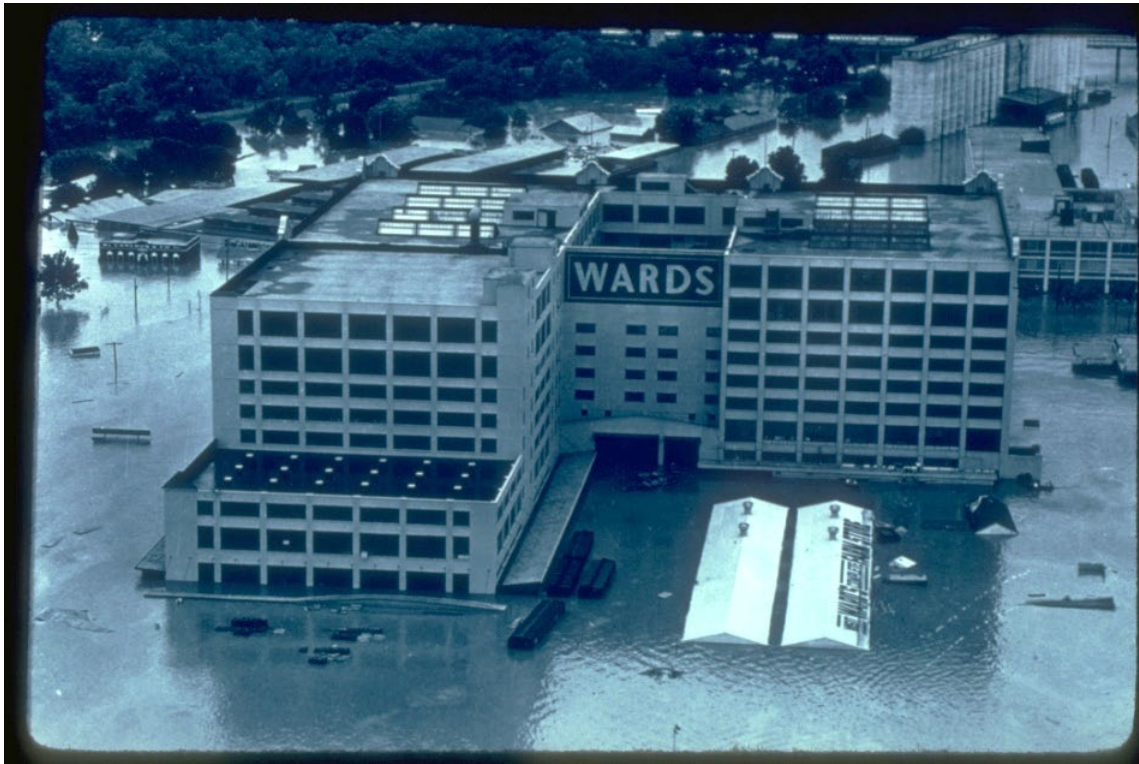
Figure 1.17: Image of Flooded Wards Building and Rooftops, Fort Worth
