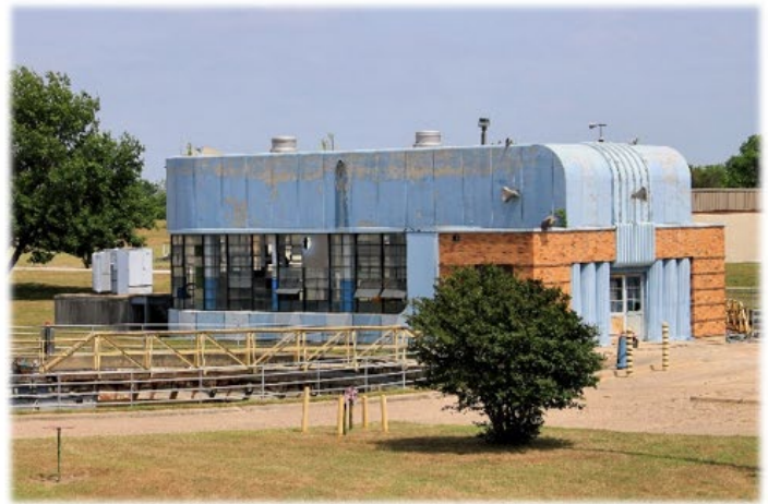
Photo of north and west side of building
