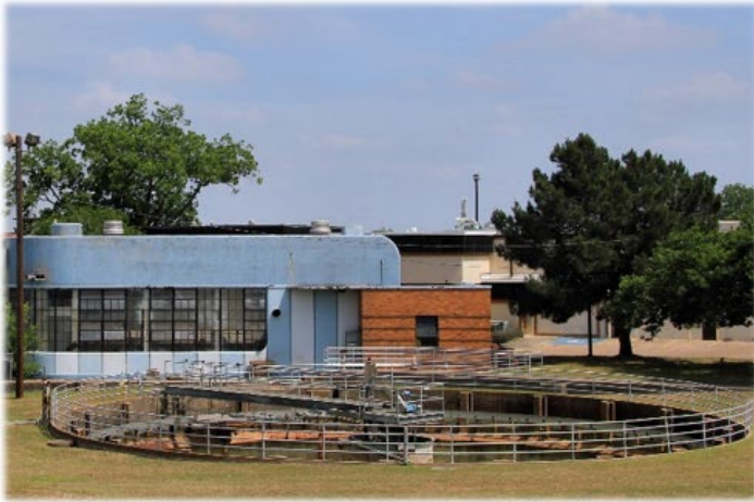
Photo of south and east side of building
