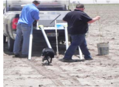
Moisture probe installation
