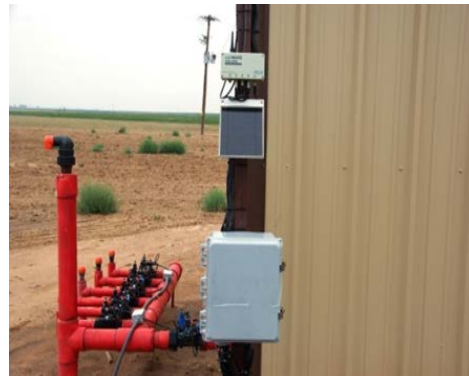
Valve bank with air relief
