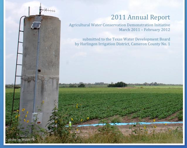
New technology adapted to a decades-old conveyance and distribution system: solar-powered telemetry system monitors and allows for remote adjustment of on-farm delivery via irrigation efficient poly-pipe in the field. HID's ADI project at work. 30 July 2012
