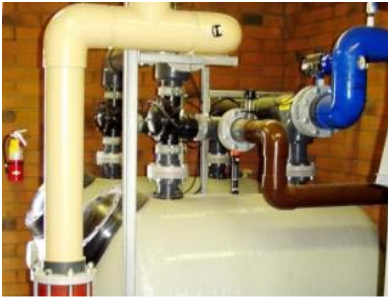
Figure 5. Large Sand Filters a Public Pool
