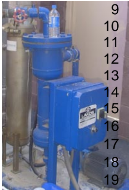
Figure 16. Cyclone Separator with Bag Filter
