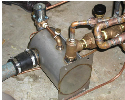
25 Figure 3. Example of a Retrofit Water Tempering Device
