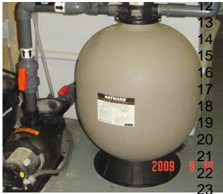
Figure 14 Typical Sand Filter
