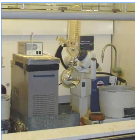
14 15 Figure 8. Recirculating Refrigeration 16 System in a Chemistry Laboratory 17
