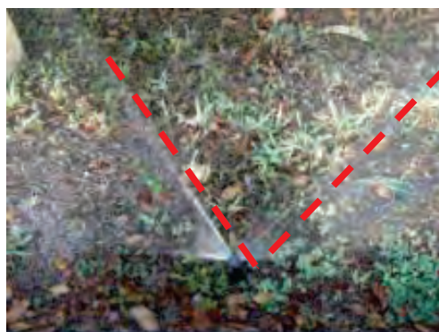
Figure 51. Clogged sprayhead, the area between the two dashed red lines is not receiving water.
