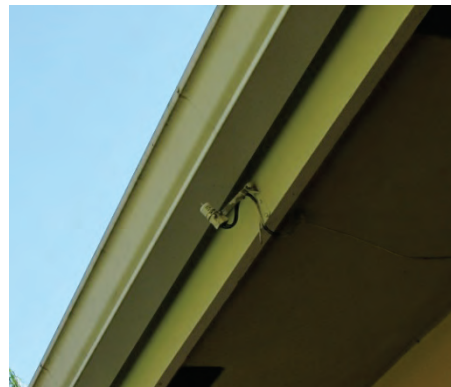
Figure 56. Rain sensors installed in places where normal rainfall is likely to be obstructed.
